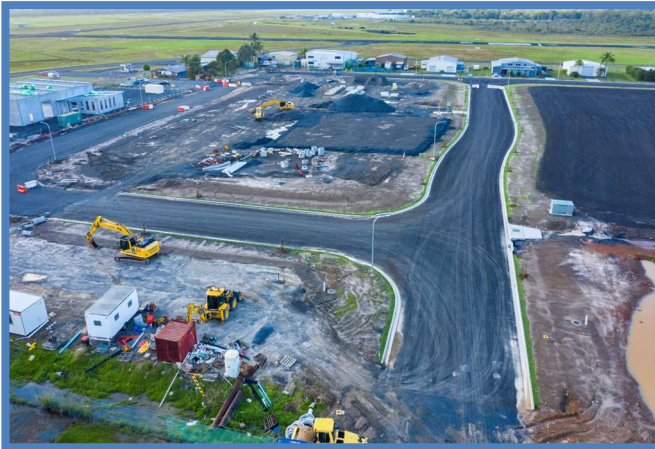
Aerial View of Works
