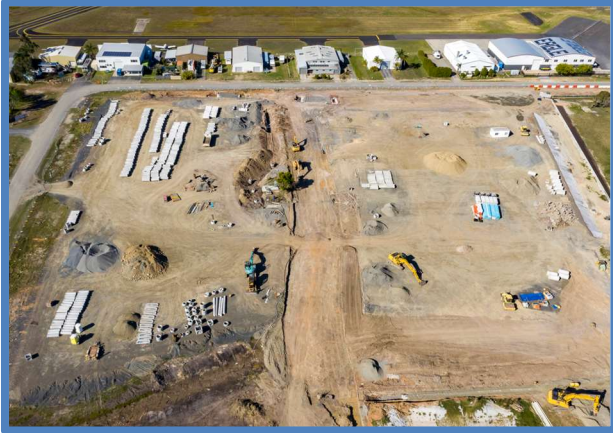
Aerial View of Works
