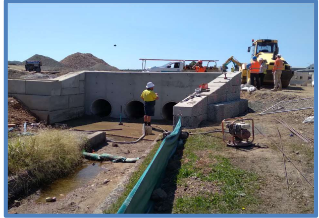
Completion of New Headwall
