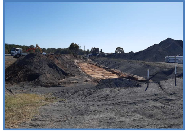
Construction Works for Road 2
