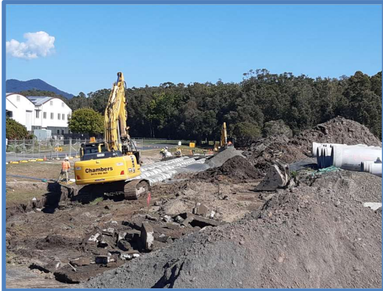
Pipe laying along Aviation Drive
